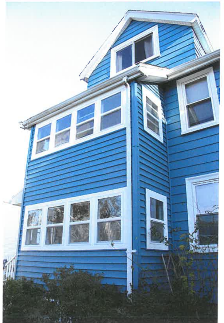
West side of house (proposed balcony location)
