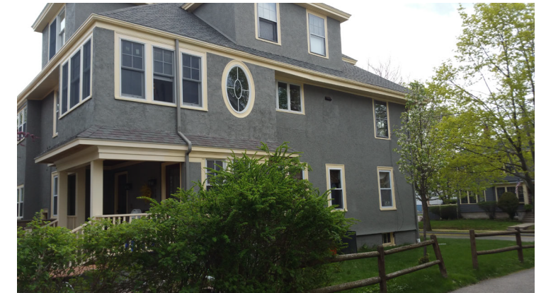
In 2010 we redesigned the delapidated rear entry to both units with a new foundation, porch, and staircase that meets current building code. We added the oval window and used double-hung windows to match the style of the house.
