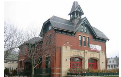
Waverley Square Fire Station
