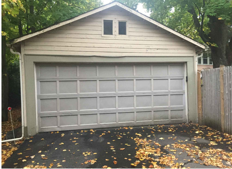
1 Garage Front Facade, view from Leonard St. NTS
