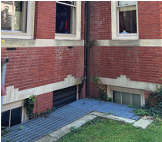
Image B-32: Grate over areaway leading to mechanical room.
