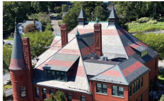
Image A-02: Aerial view of the polychromatic slate roof featuring copper crenelated cresting, turrets, and cupolas.
