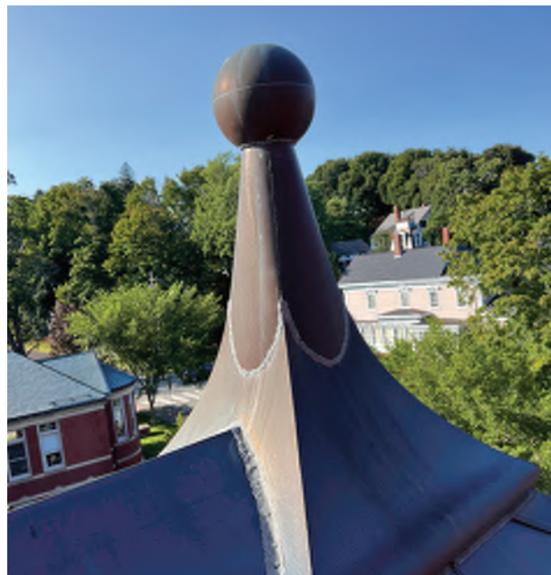
Image C-09: The rilled copper at ridge caps and finials are intact and in good shape..
