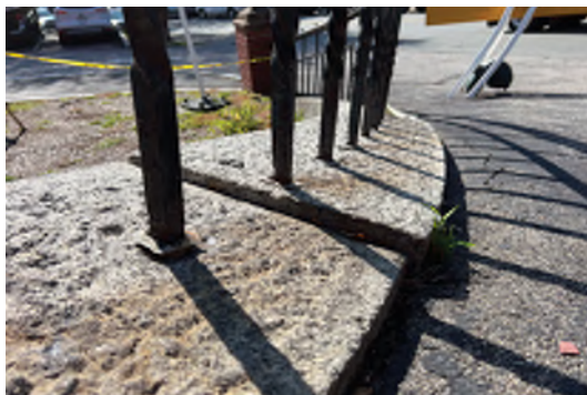
Image A-58: Original metal handrails embedded in the granite coping stones at the south retaining wall.
