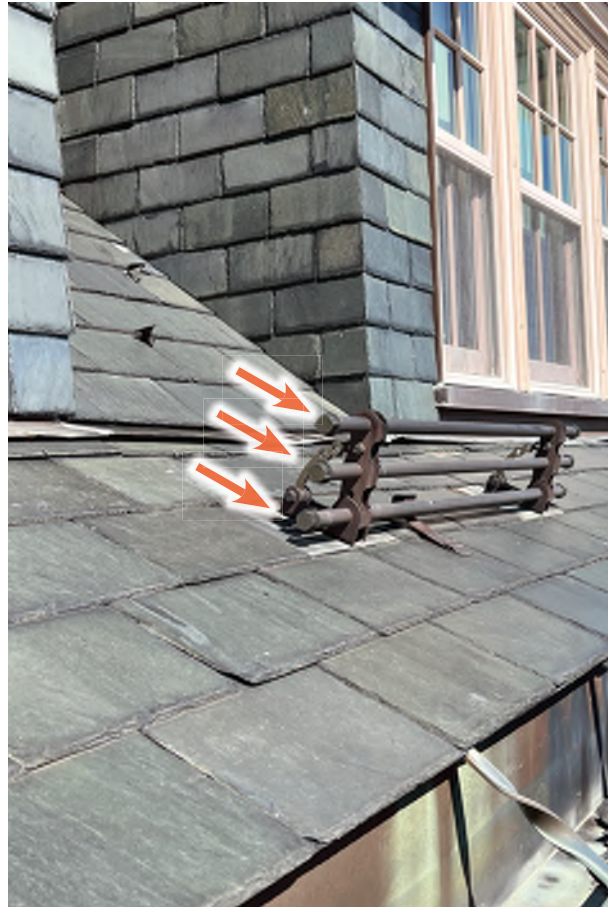
Image C-17: The 3-pipe snowguard fences can be easily detached without removing their brackets.
