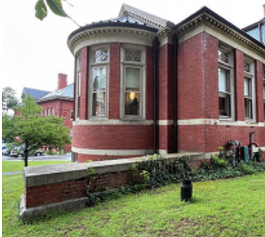
Image B-28: Severely deteriorated north site wall caused by water infiltration through sky-facing joints.
