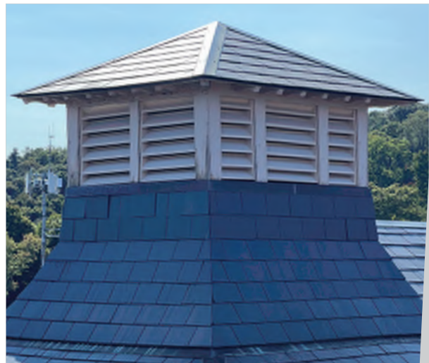
Image C-02: A pair of slate-clad ventilators adorn the main ridge.
