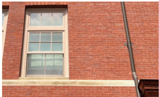
Image C-47: Overall, the building benefits from well-maintained masonry, all in excellent condition.
