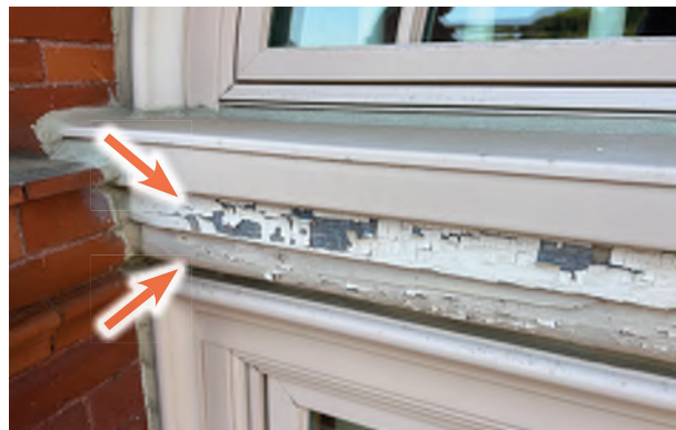
Image C-41: Though small, the remaining window wood transoms should be cared for and repainted.
