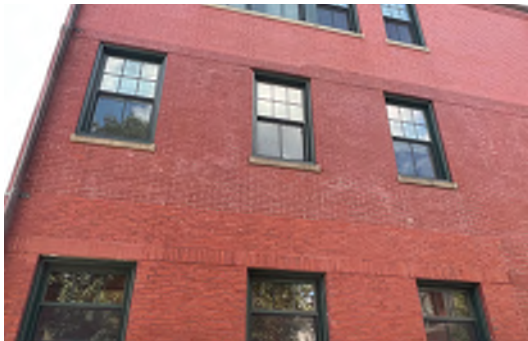
Image A-35: View of the north elevation of the Town Hall addition showing the three different brick colors.
