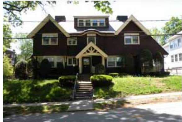
15 Lawndale Street (also above) prior to demolition, 2009 (Michael Smith)
