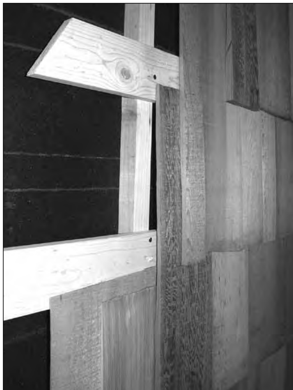
Figure 8. Rain screen technique.
