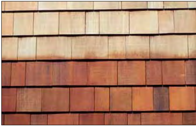
Figure 14. Semitransparent stain application to shingles that were let weather for about two years. NOTE: The stain application was not done correctly. The painter allowed stain to partially coat the bottom of the course of shingles directly above the stained portion. When the shingles above are stained, there will be a lap mark.
