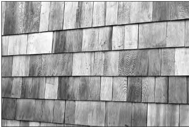
Figure 5. Newly installed shingle siding with transparent water-repellent preservative finish.
