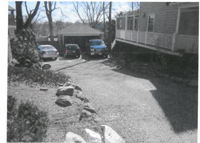
EXISTING DRIVEWAY WIDTH IS TOO NARROW FOR SHARED EASEMENT WITH NEIGHBOR ESPECIALLY WHEN BACKING UP TO BUSY PLEASANT STREET. EXISTING STONE WALL HAS BEEN HIT OVER A DOZEN TIMES DURING THE LAST YEAR BY GUESTS.
