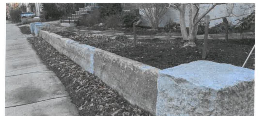
RECLAIMED GRANITE CURB AS RETAINING WALL
