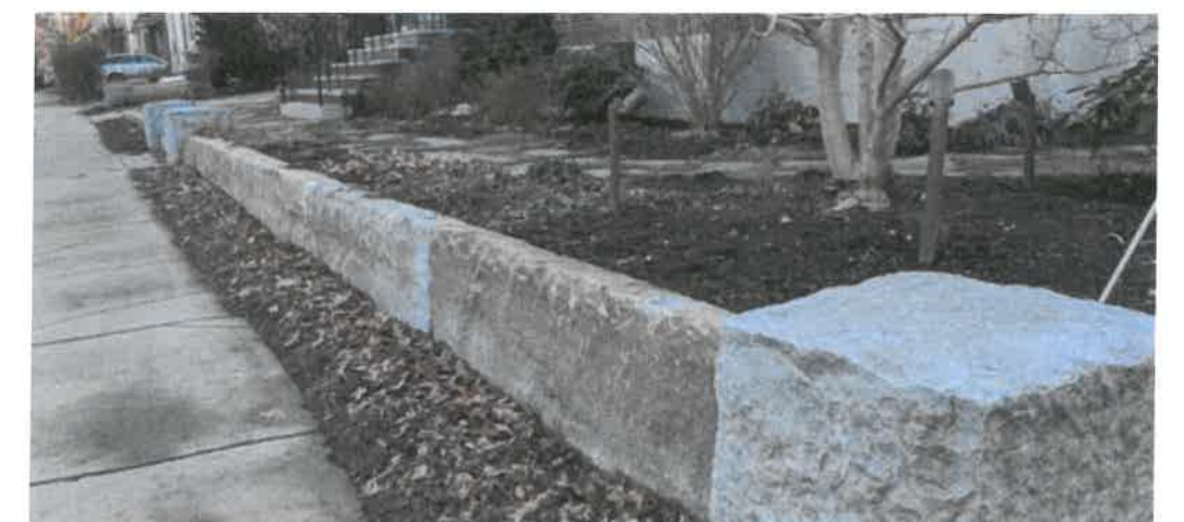
RECLAIMED GRANITE CURB AS RETAINING WALL
