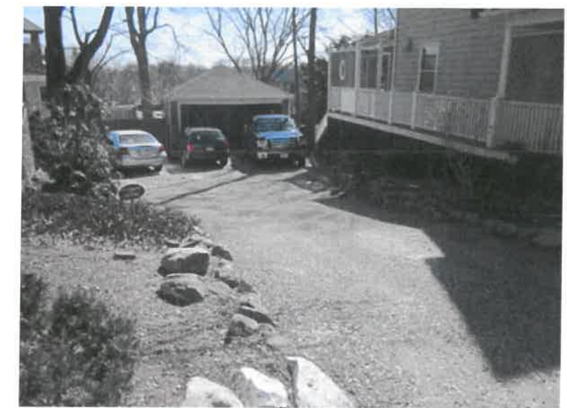
EXISTING DRIVEWAY WIDTH IS TOO NARROW FOR SHARED EASEMENT WITH NEIGHBOR ESPECIALLY WHEN BACKING UP TO BUSY PLEASANT STREET. EXISTING STONE WALL HAS BEEN HIT OVER A DOZEN TIMES DURING THE LAST YEAR BY GUESTS.
