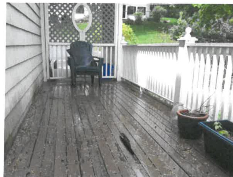
EXISTING DECK IS CRACKED, ROTTING AND UNSAFE WHILE SITUATED IN AN UNDESIRABLE LOCATION. TO THE NORTH IT GETS NO SUN AND IS PRONE TO MILDEW. WHILE DECK HAS NO PRIVACY AND IS CONSTANTLY EXPOSED TO THE LOUD TRAFFIC OF PLEASANT STREET.
