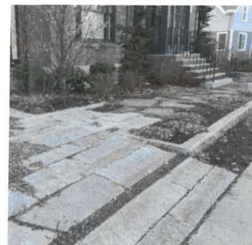
RECLAIMED GRANITE CURB AS LANDING
