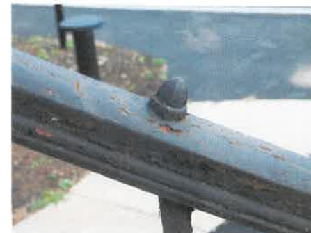
5 Existing Top Rail Photo 12" = 1'-0"
