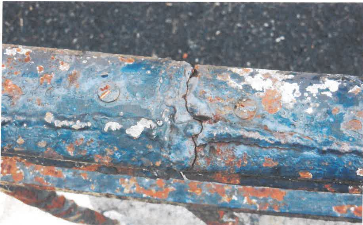
4. Close up view of top rails showing both welds and screws.
