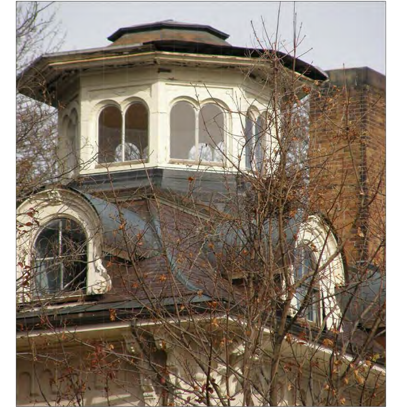
VIEW OF EXISTING CUPOLA
