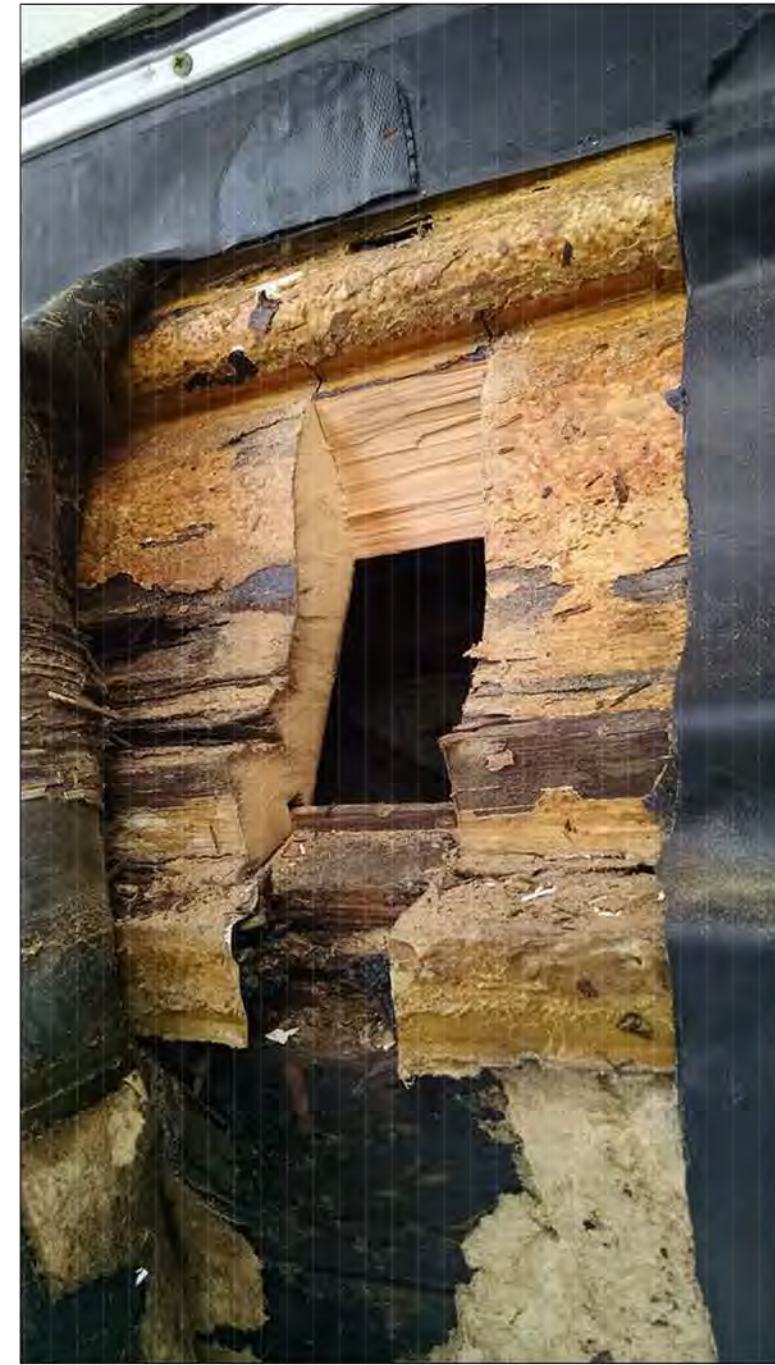
WOOD-BASE MOLDING UNDER ROOF MEMBRANE BELOW CUPOLA
