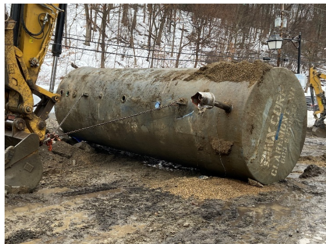
Service station tank removal
