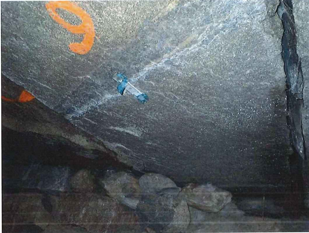
Photo 7: Typical underside, granite slab looking east.
