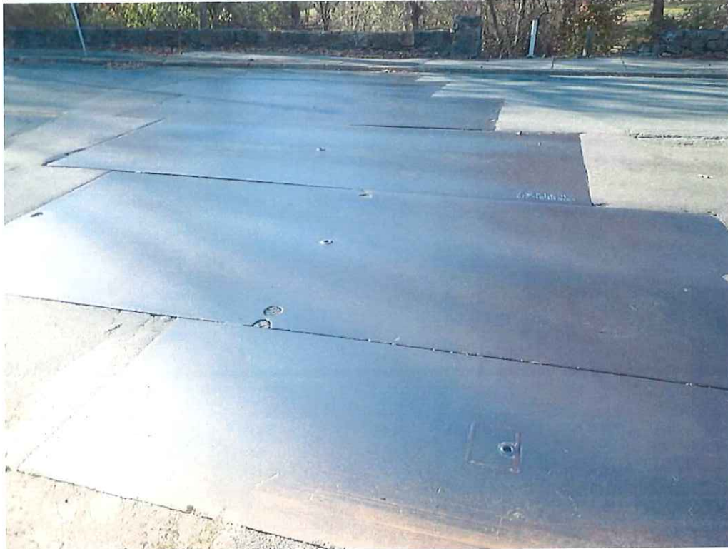
Photo 11: Typical retrofitted steel roadway plates looking south.
