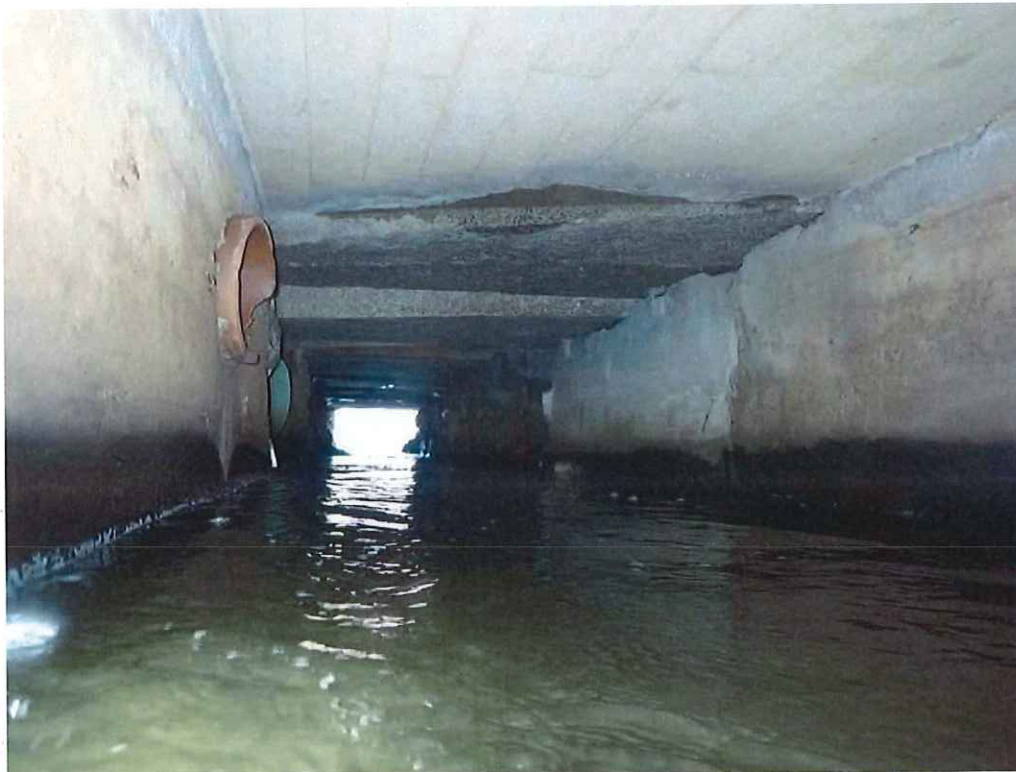
Photo 10: Typical underside, concrete extension looking south.
