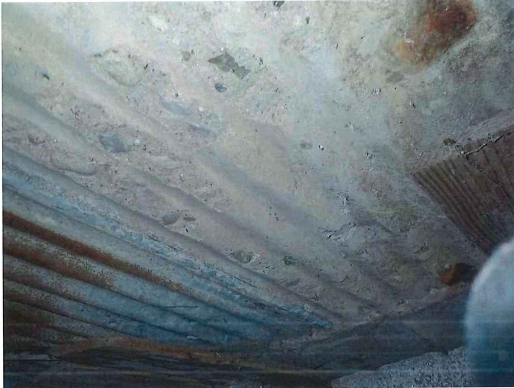
Photo 9: Typical underside, concrete slab looking west.
