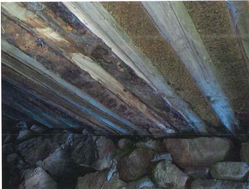
Photo 8: Typical underside, steel beams looking east.
