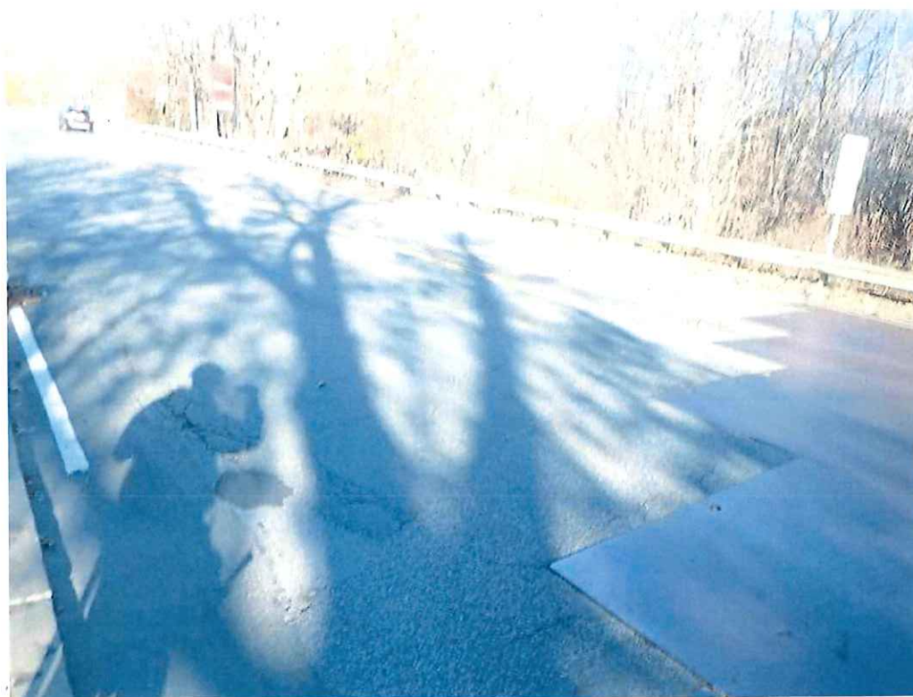
Photo 2: West approach, looking west.
