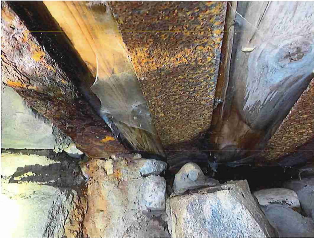
Photo 7: Heavy section loss up to 100% at the west end of the bottom flanges of beams 6-8.
