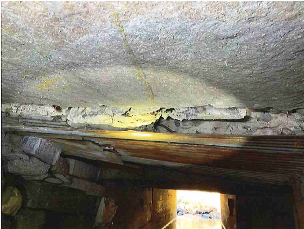
Photo 8: Reinforced concrete slab, There are two spalls with exposed rebar along the south edge measuring up to 2'-6" long x 9" high x 6" wide.
