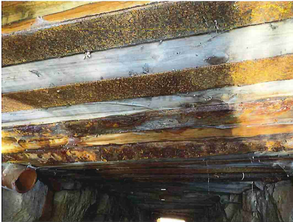
Photo 5: The beams typically exhibit minor rotation about the longitudinal axis, resulting in the bottom flanges no longer being level (Note the timber shielding in between beams).
