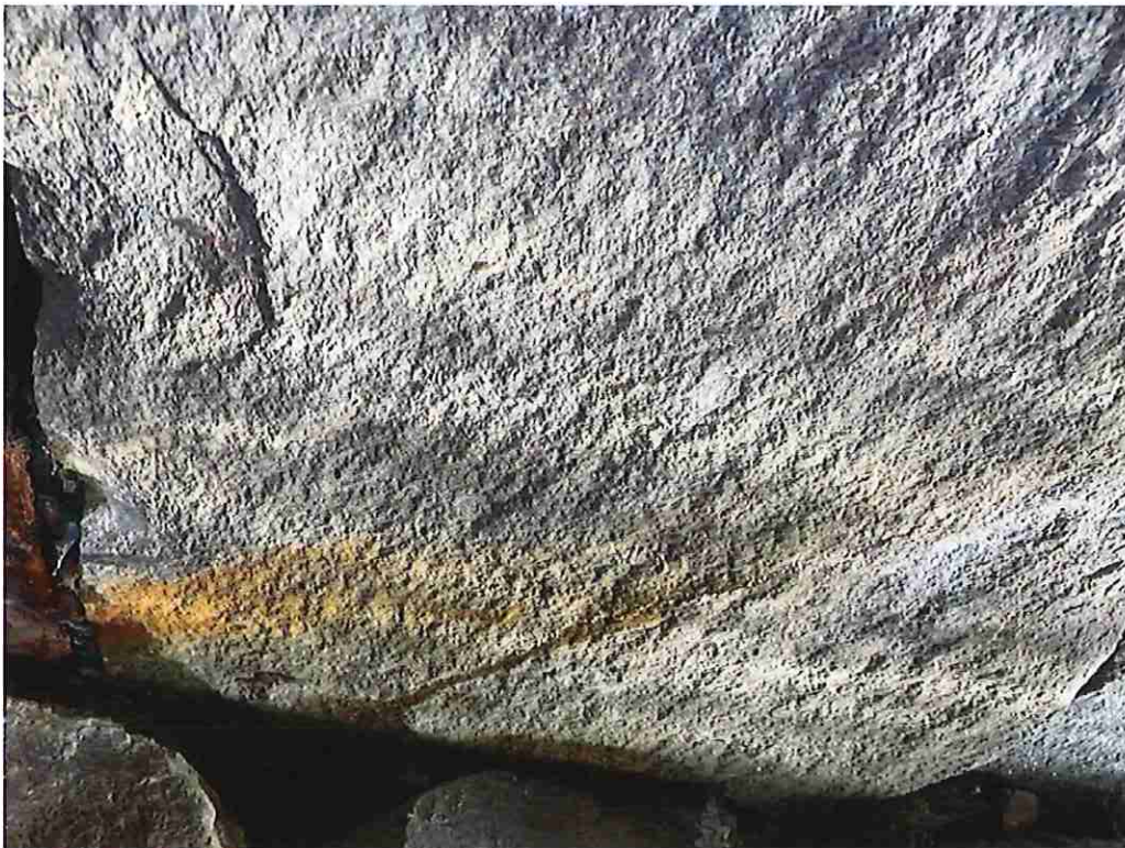
Photo 2: Granite Slab 4, there is a diagonal hairline crack at the east end.
