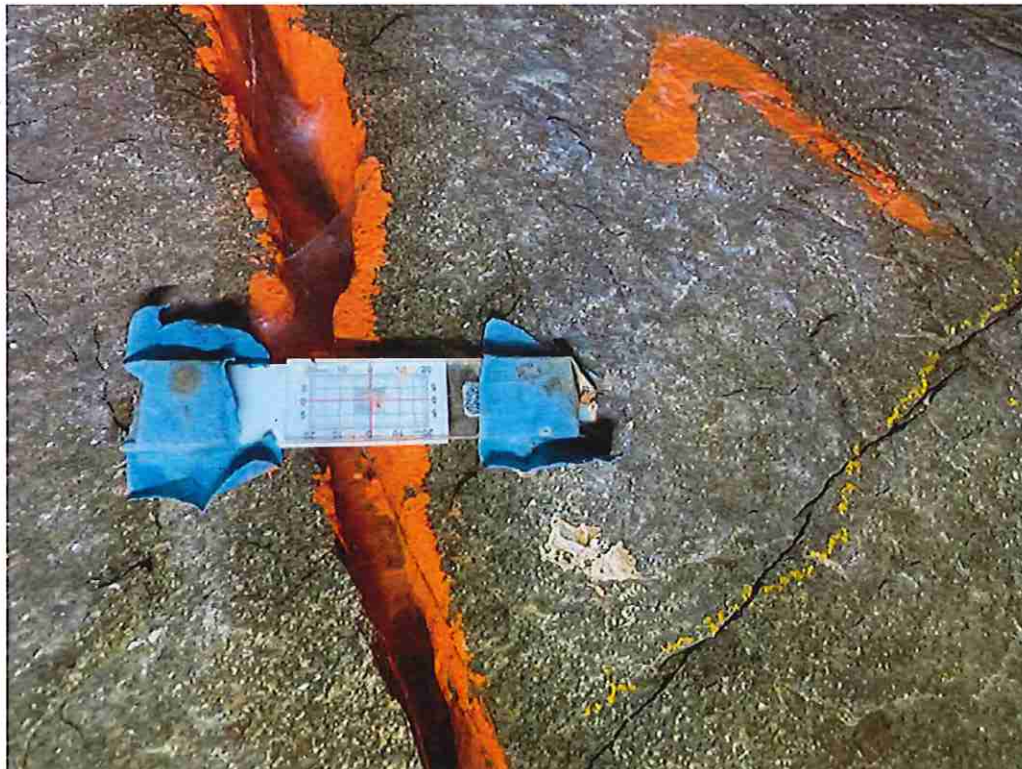
Photo 4: Granite Slab 7 crack monitor installed reading 0.05 mm of movement, there has been no change since the previous inspection.
