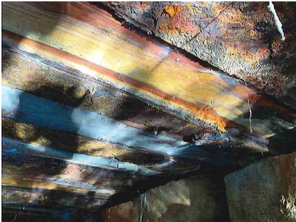
Photo 6: Heavy section loss up to 100% at the east end bottom flanges of beams 7-8.
