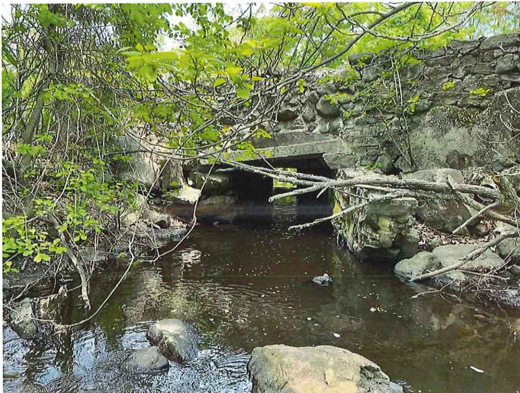
Photo 4: Typical South Elevation
