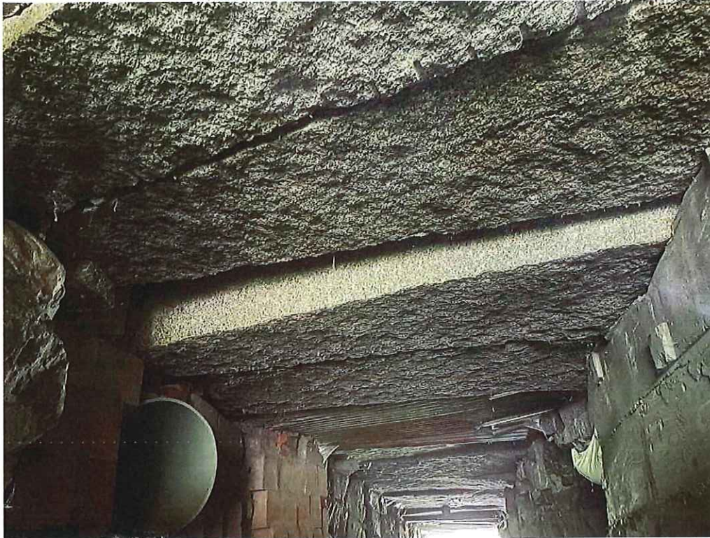
Photo 7: Typical Underside looking south
