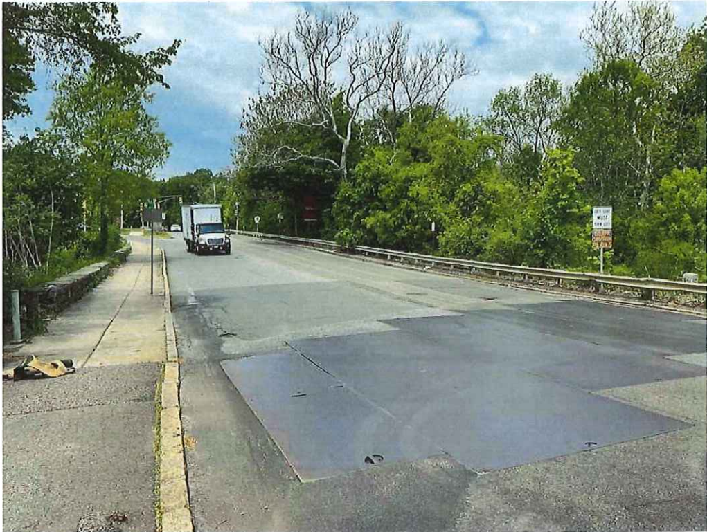
Photo 1: Typical East Approach looking west
