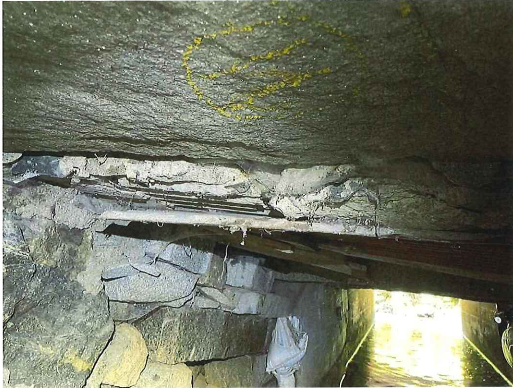
Photo 23: Concrete slab at the south edge: Two (2) up to 2'-6" L x 6" W x up to 9" D spalls with exposed rebar.
