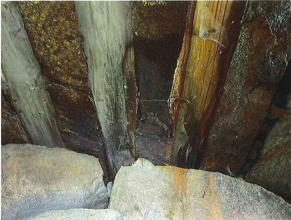
Photo 15: Steel Beam 2 bottom flange at West Abutment: 100% section loss x 1" wide at the south toe with 3/16" thickness remaining.
