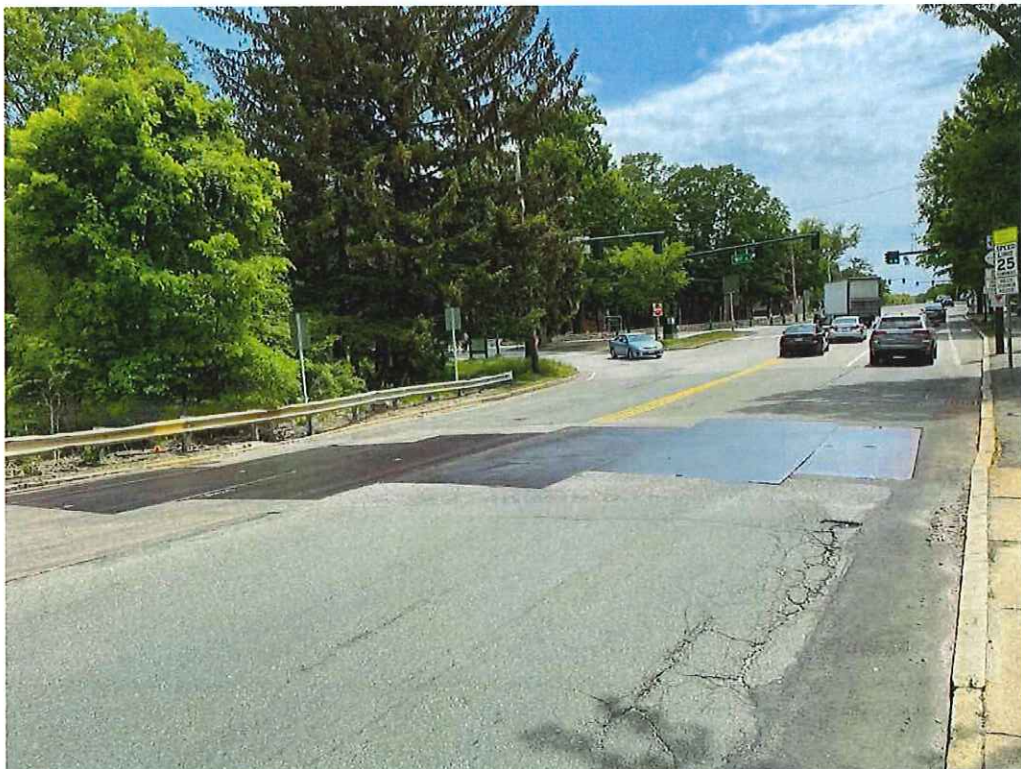
Photo 2: Typical West Approach looking east
