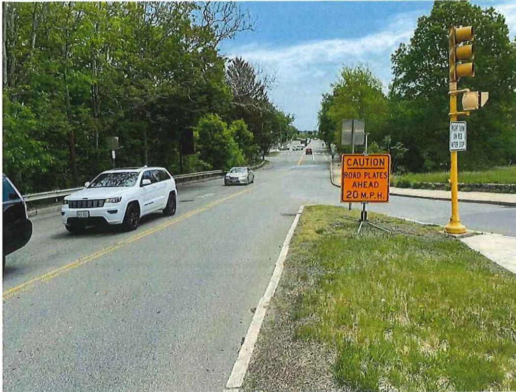
Photo 9: "Caution" sign in-place at the west approach
