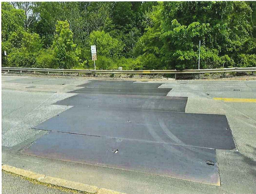
Photo 10: Typical retrofitted steel roadway plates looking north.
