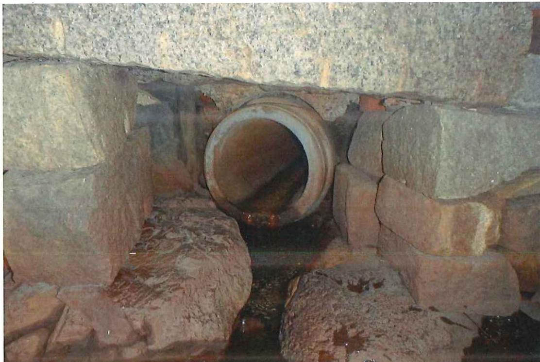
Photo 16: West breastwall: Drainage opening adjacent to wall repair.
