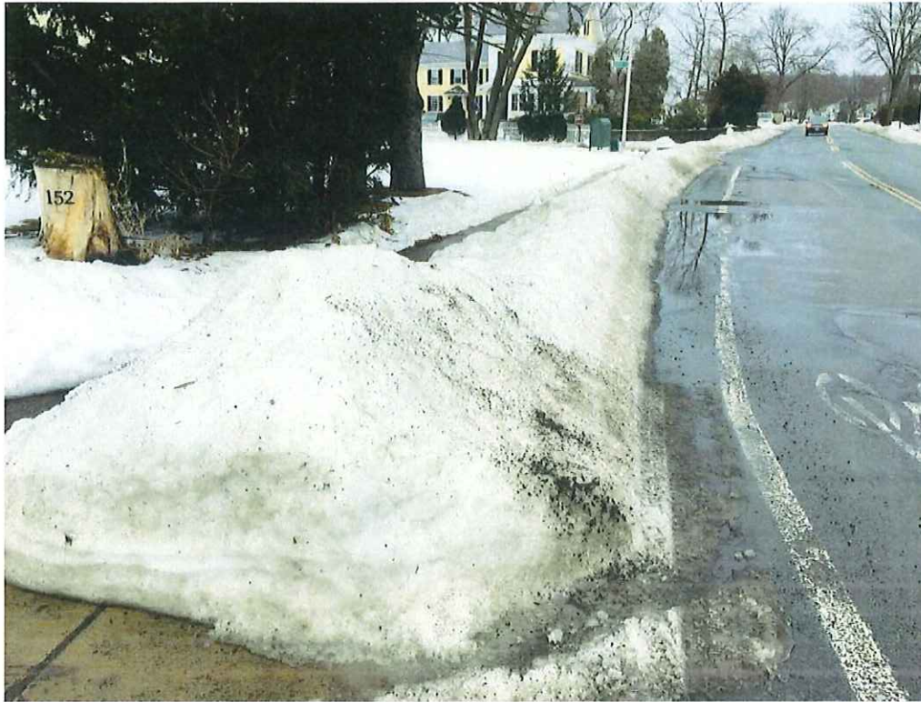
Photo 17: Sidewalks were covered by snow at the time of the inspection.
