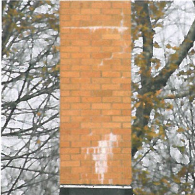
Brick replacement and repair
