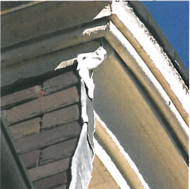
Exposed slate at edge detail
