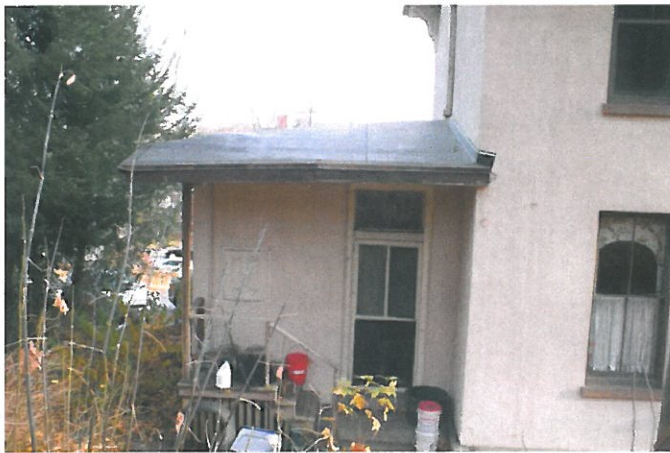
4. Ice chest stairs and roof extension framing materials not in historic context.
