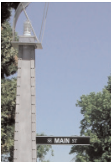
Lighting on Eastbank Esplanade. Portland, OR
