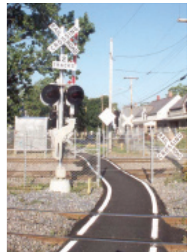
Dual track grade crossing. Burlington, VT
