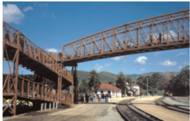
Trail-rail overcrossing. San Luis Obispo, CA
