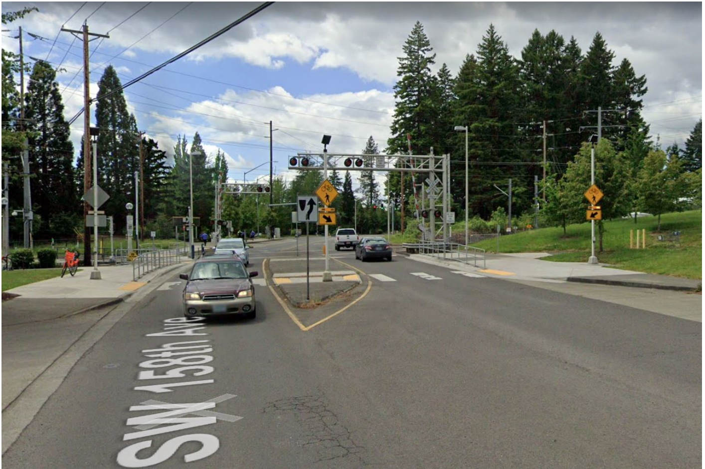
Rail with trail crossing with RRFB, 1797 SW 158th Ave, Beaverton, Oregon
