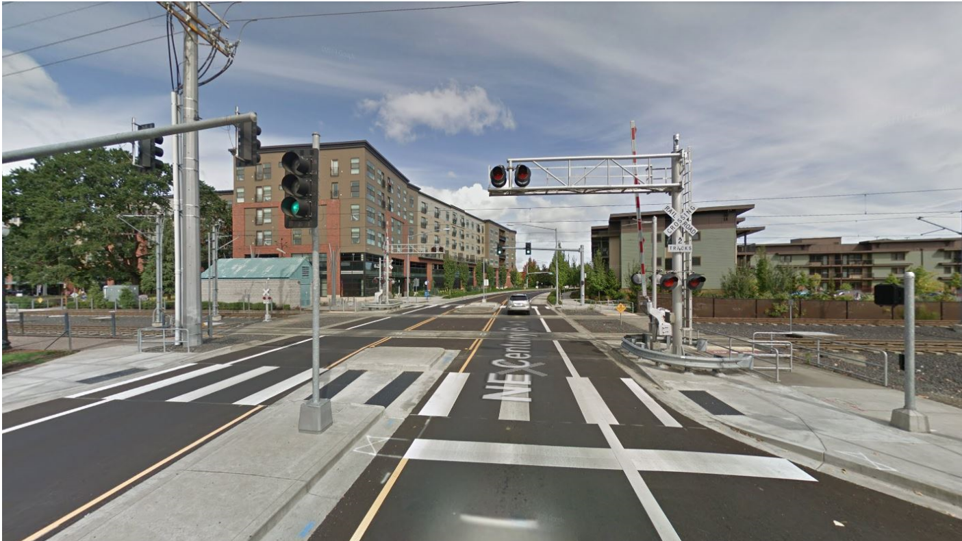
Midblock Traffic Signal adjacent to Railroad Crossing, 1401 NB 231st Avenue Hillsboro Oregon
