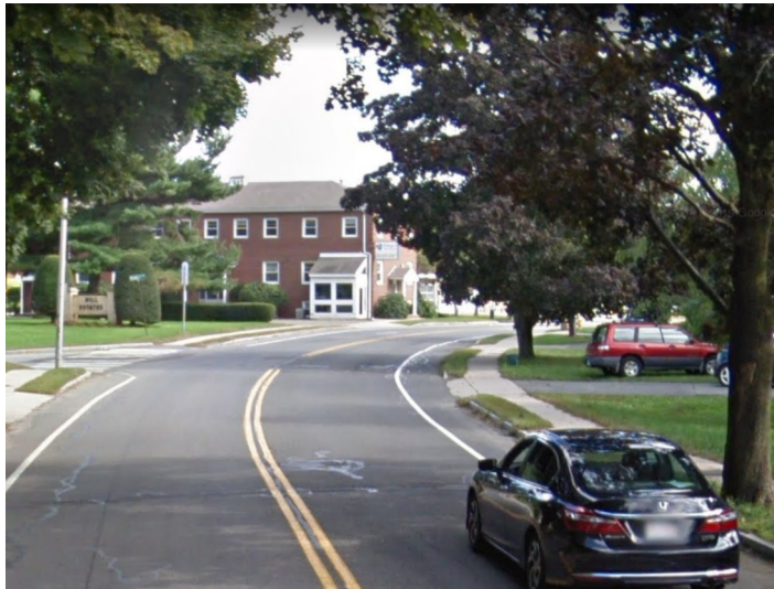
Looking southbound approaching Pond Road, the roadway curvature contributes to the poor visibility of queuing traffic at the Railroad Crossing
