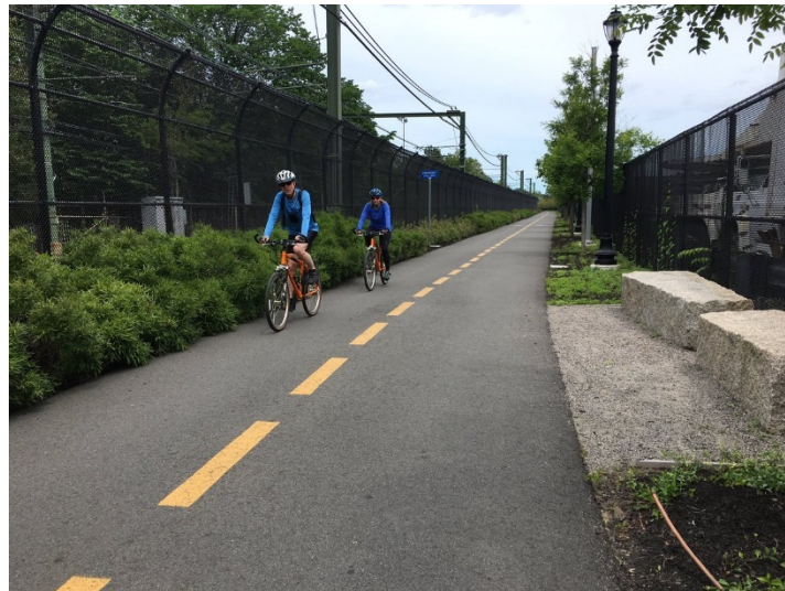
Chain Link Fence Between East Boston Greenway and MBTA Blue Line
