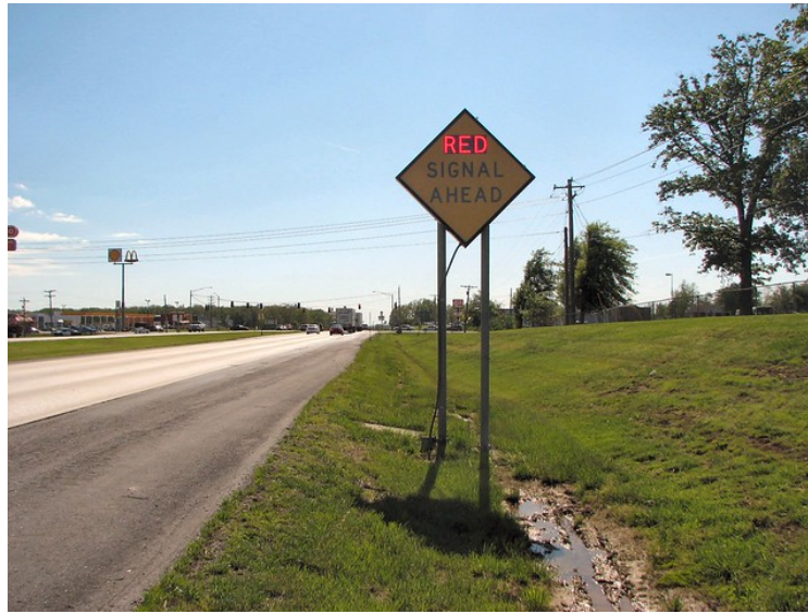
Example of Advanced “Red” Signal Ahead” activated bank-out sign Assembly
