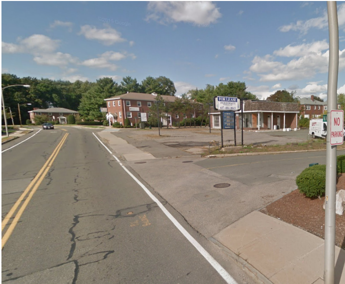
No Stop Sign or Stop Bar for side street approaches
