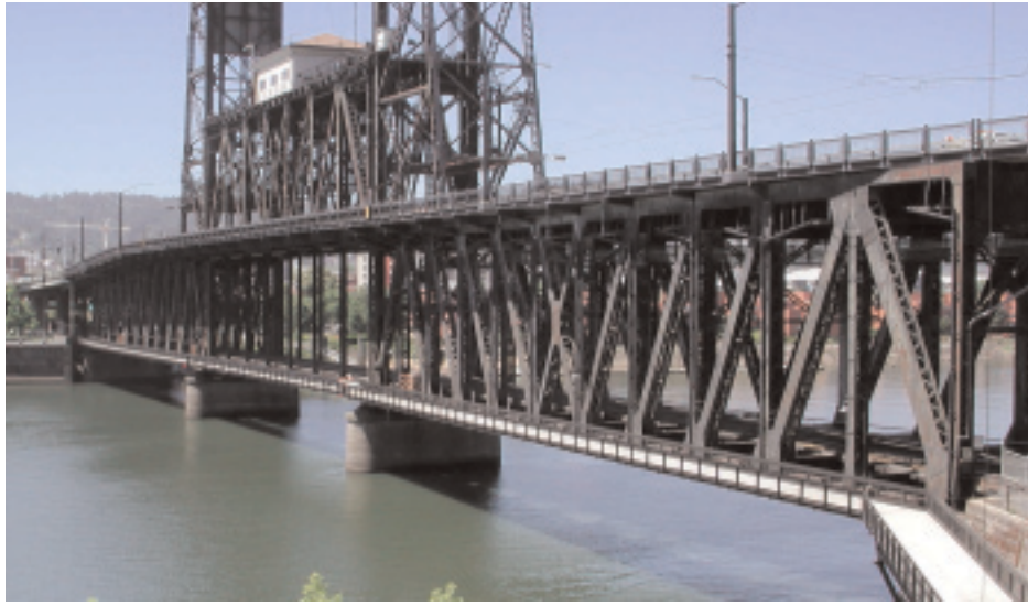
Steel Bridge Riverwalk. Portland, OR
