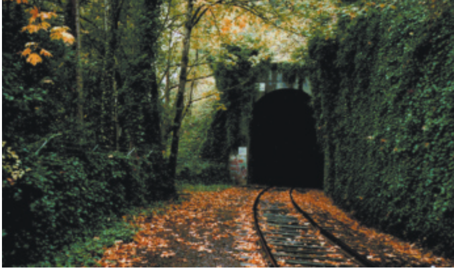
Single track tunnel on Lake Oswego Trolley Line. Lake Oswego, OR
