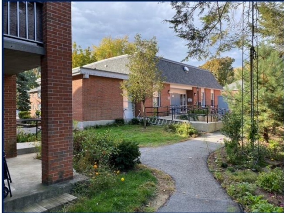
Sherman Garden's community building is well-used, but in deteriorating condition
