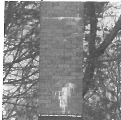
Brick replacement and repair
