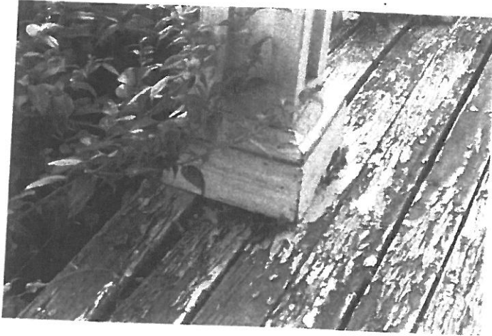
9. Front west piazza column bases.
