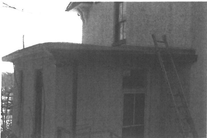
20. Access setup to review opening at edge of roof over ice chest entry.
