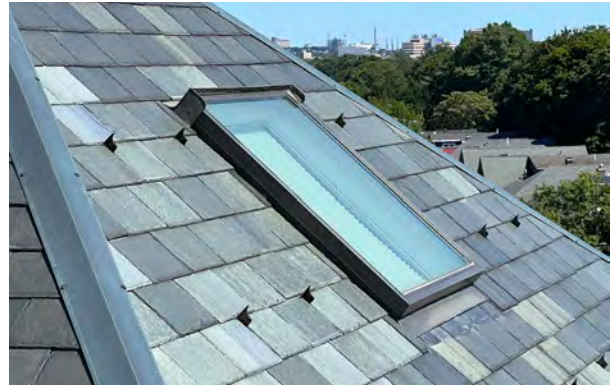
Image C-11: Modern skylight punctuate the slate roof in a few locations, with no reported leaking..
