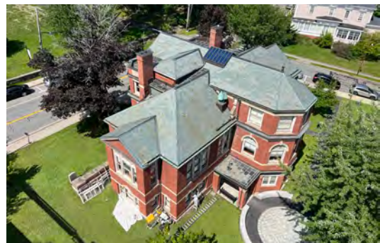
Image B-02: Aerial view of the School Administration Building from the southeast.
