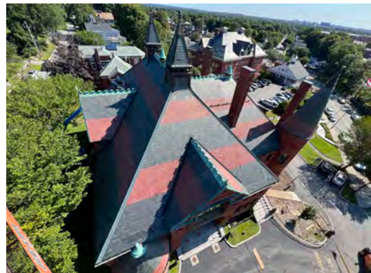
Image A-03: Aerial view of the roof showing recently replaced hip caps and valley flashing.
