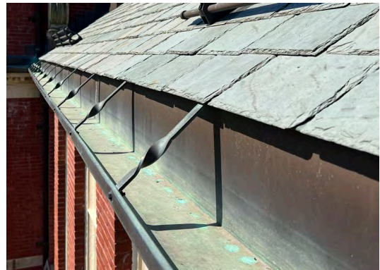
Image B-16: Approx 20 year old copper downspouts in good condition. No corrosion, pinholes, or metal deterioration.
