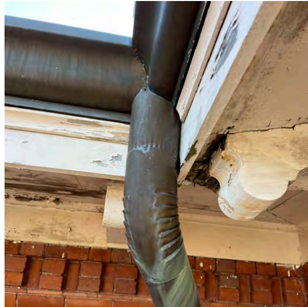
Image C-26: Copper downspout elbows are intact and appear to perform as they should.
