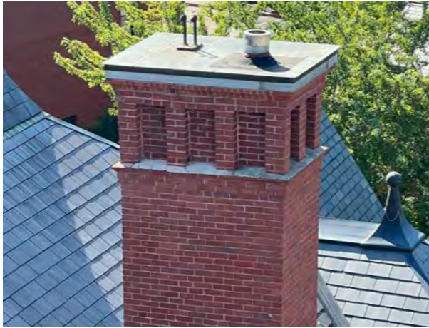
Image C-43: The building's solid brick chimney is plumb and intact, and appears to be well-capped.
