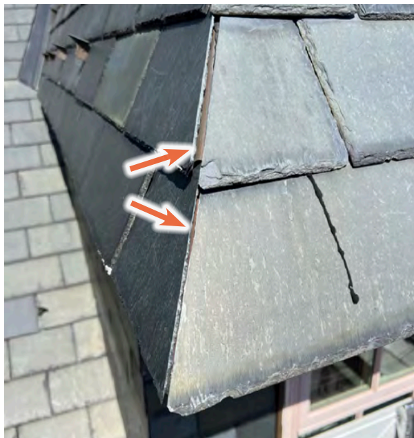
Image C-08: Interwoven flashing between the slate courses on the dutch gable dormer is a quality detail and water-resistant.
