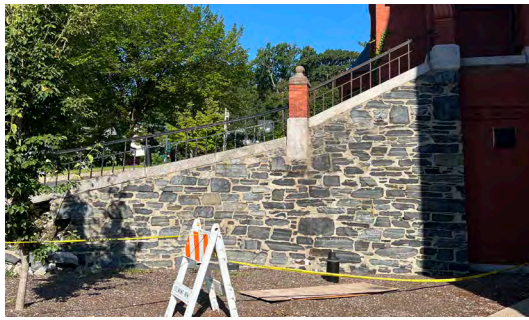
Image A-56: View of the cheek wall at the south portico integrated with the retaining wall.
