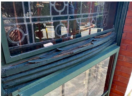
Image A-45: Spalling at brick masonry below the cracked first floor cast stone window sills at the north elevation.
