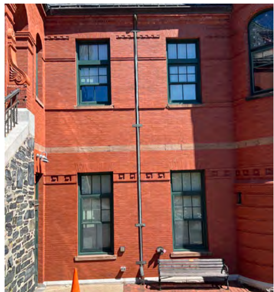
Image A-20: View of inset copper gutters at the south elevation. Copper gutters typically drain into cast iron boots.
