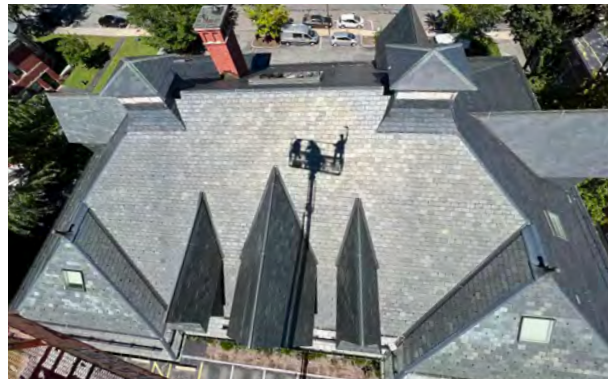
Image C-01: The Homer Building is comprised entirely of black slate in at least two textural varieties.
