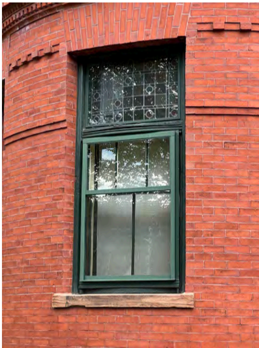
Image A-44: View of original wood window at south projecting window bay with stained glass transom.
