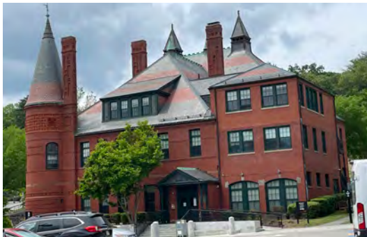
Image A-43: View of the east elevation where showing the various types of new aluminum windows on the building.
