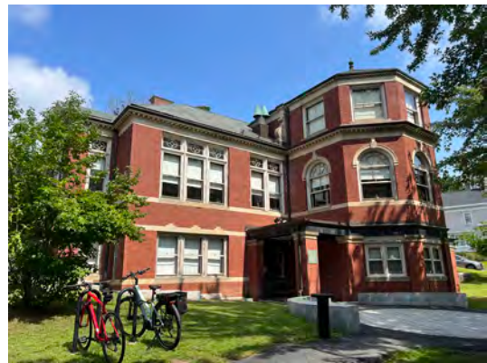
Image B-29: View of the southeast corner of the building showing various types of original and new windows
