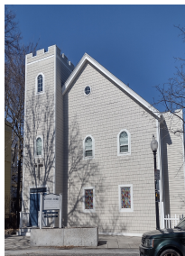
Cambridge Western Ave Baptist Church 299 Western Ave Proj 22-5 $13,500 Roof Complete
