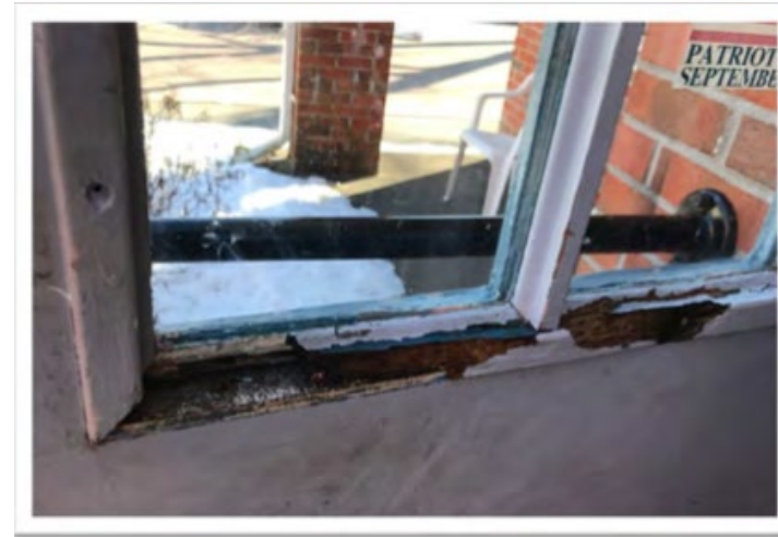
Rust and failing joint sealant
