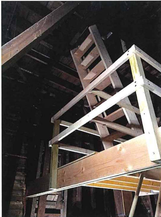
Figure 4- New ladder to clock movement
