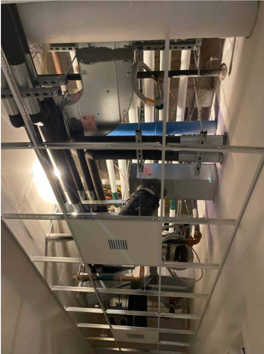
Area F Level 1 Above Ceiling
