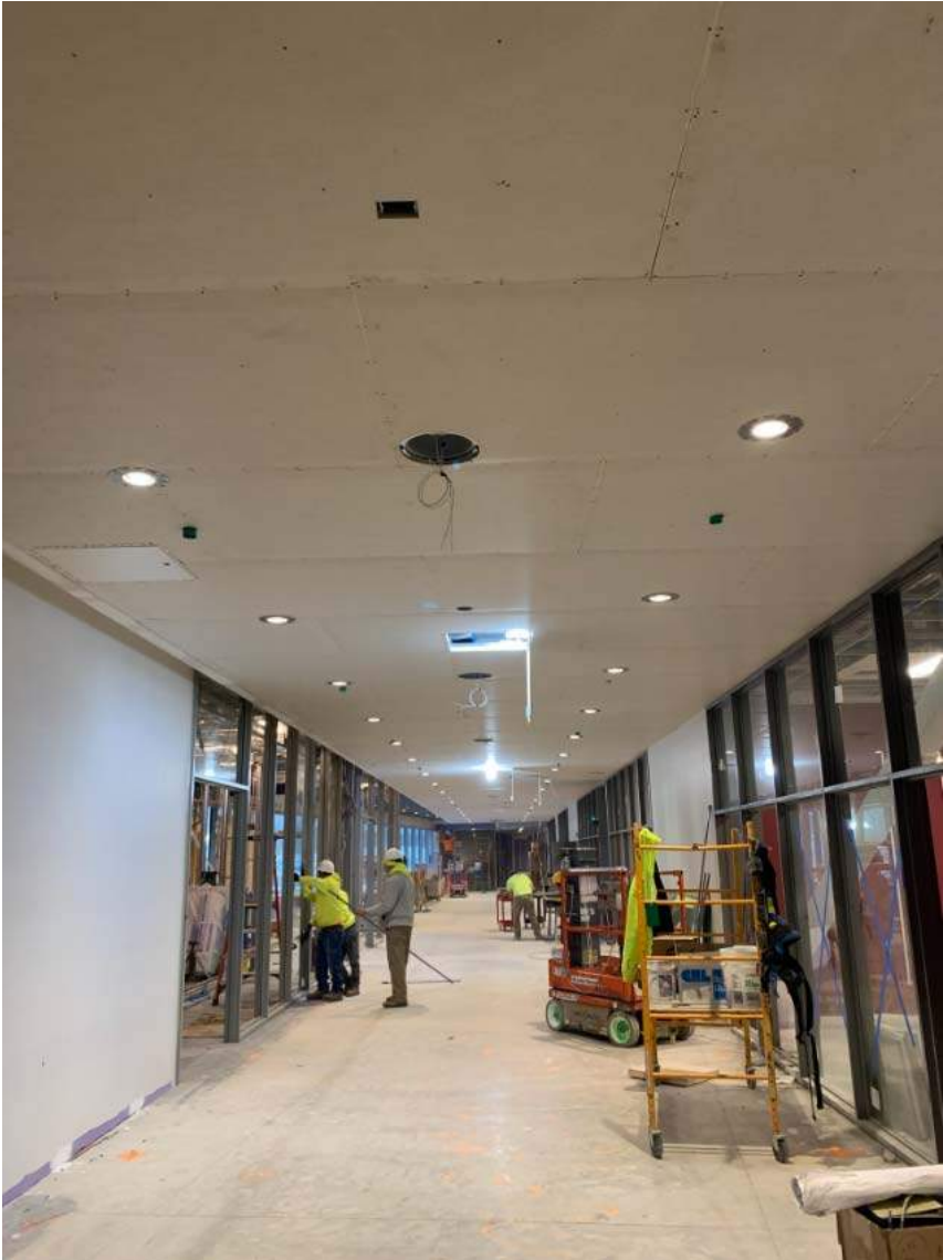
Area D Level 1 Corridor
