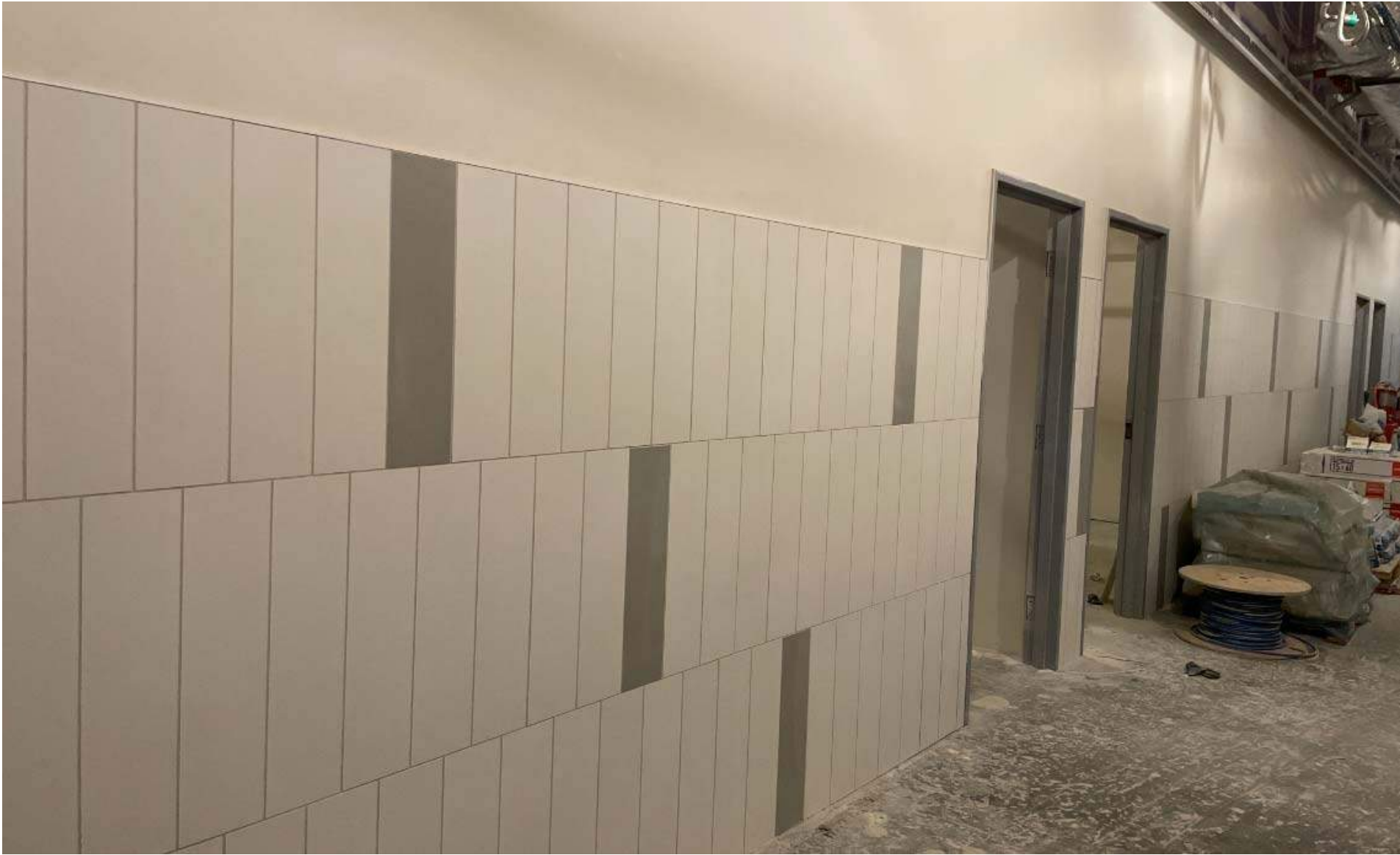
Area F Level 1 Corridor
