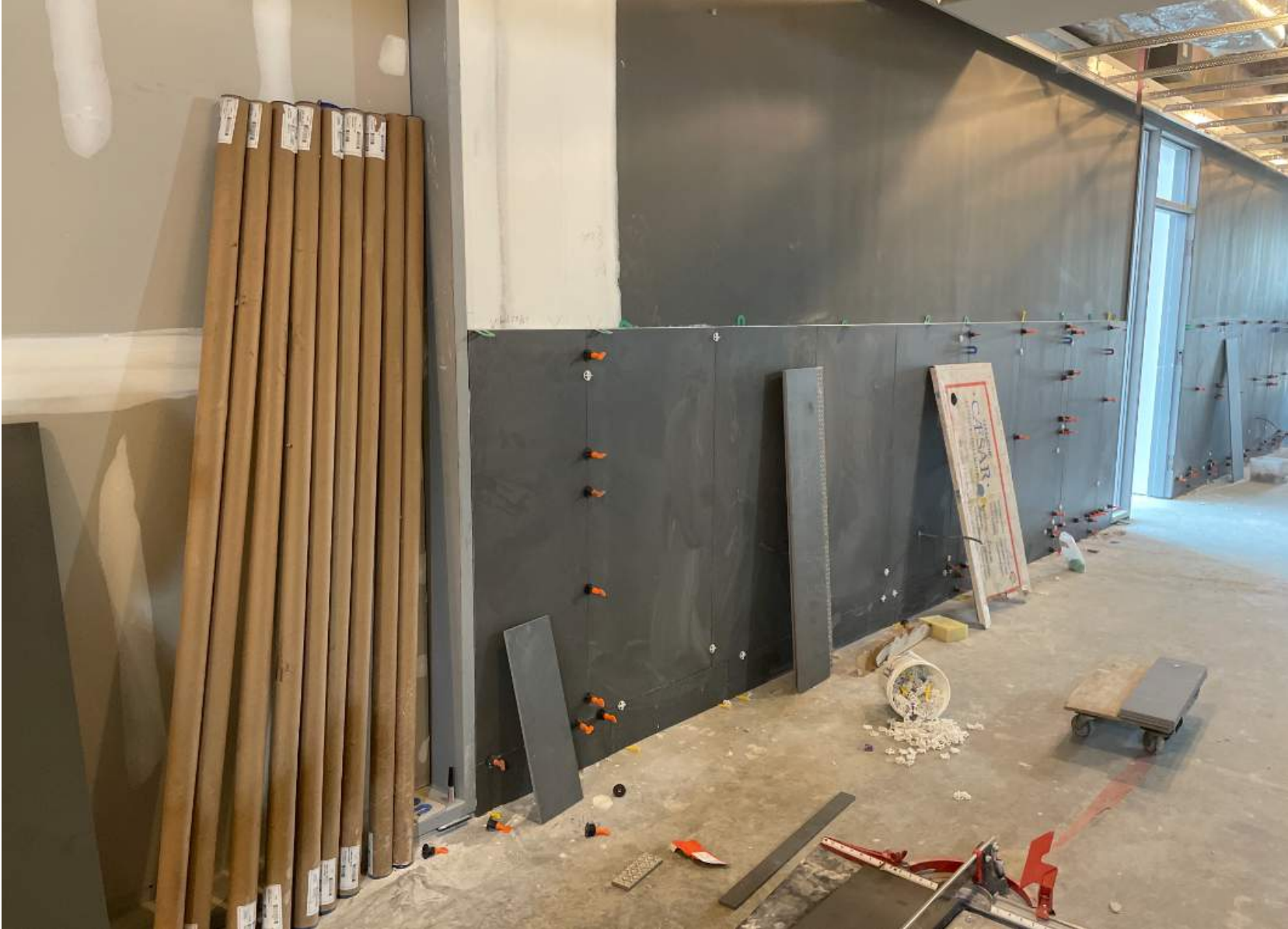
Wall Tile Install
