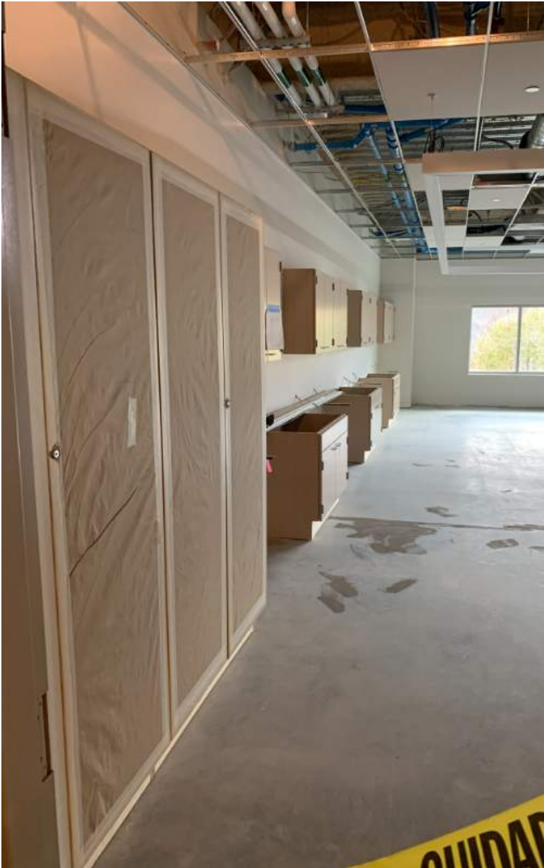
Casework and Flooring Prep
