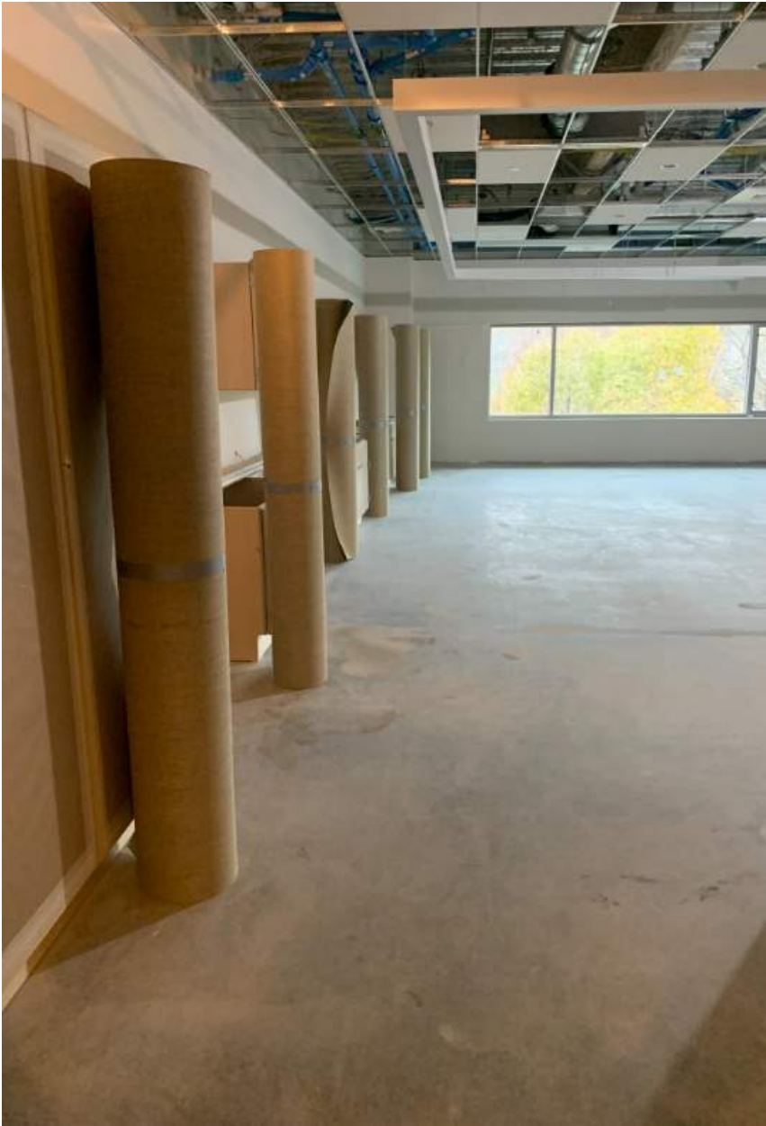
Linoleum Flooring Prep
