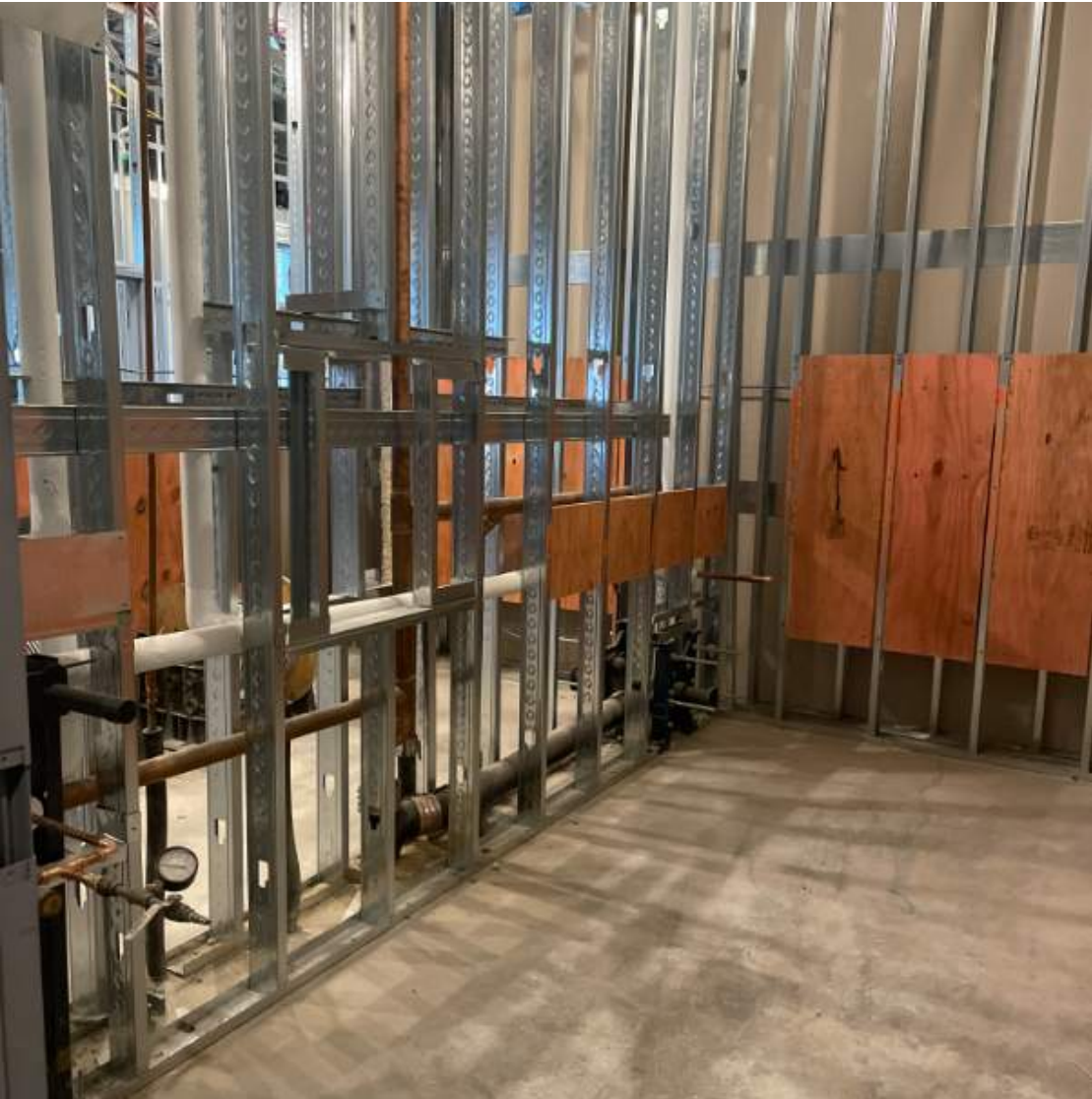
Bathroom In-wall Rough-in and Blocking
