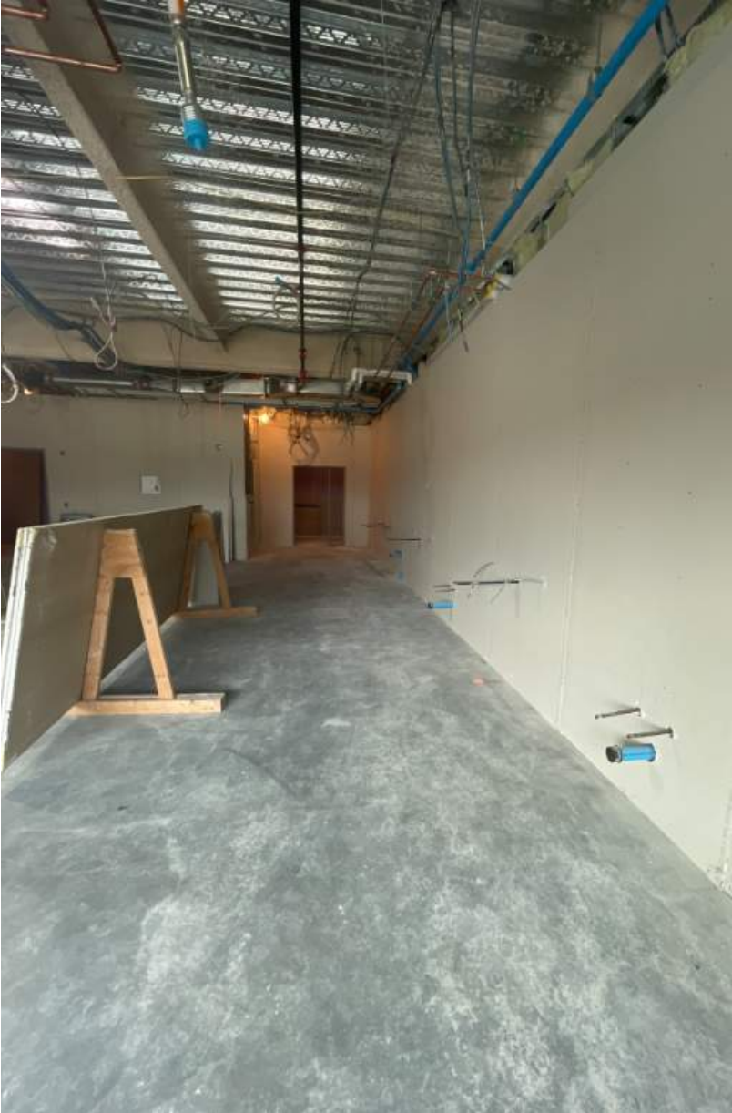
Plumbing Rough-in and Drywall
