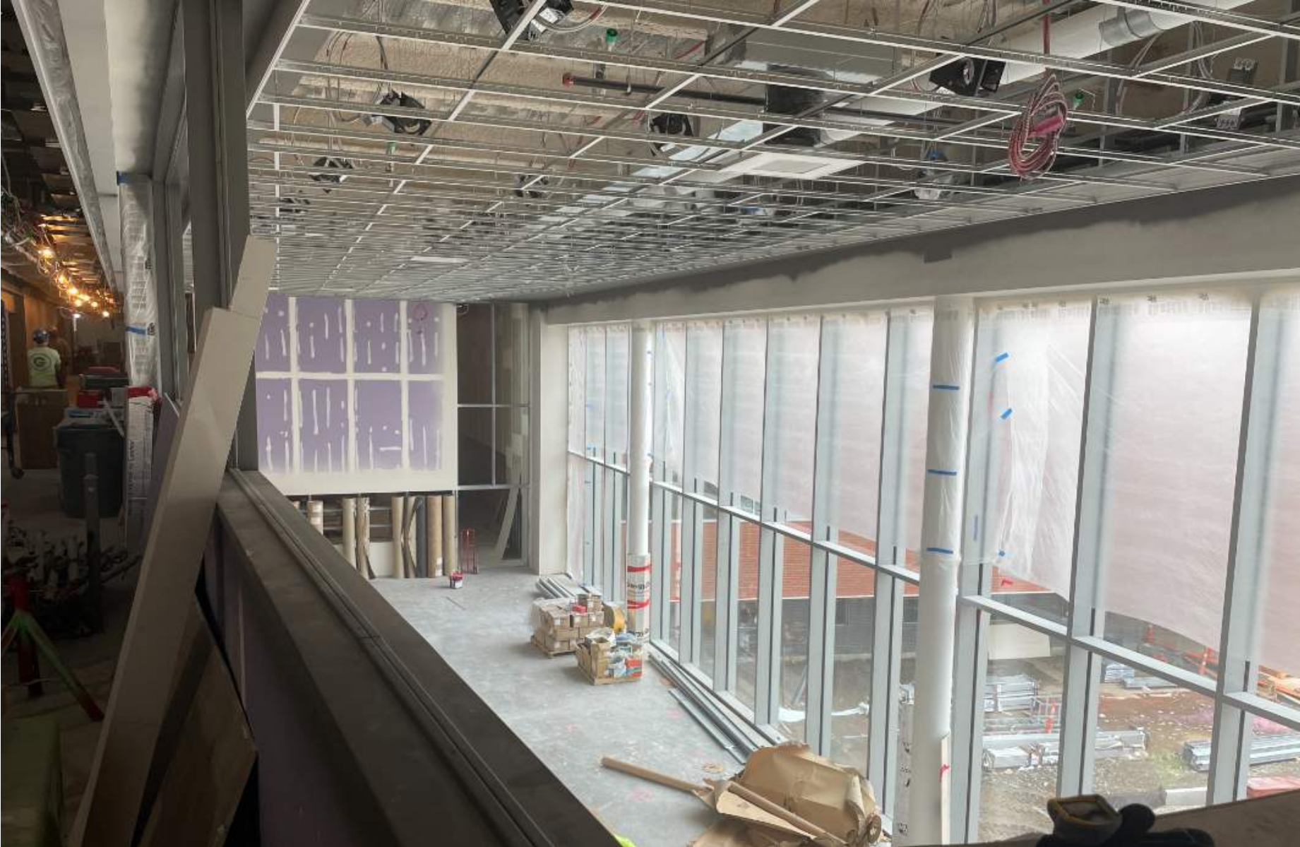
ACT Ceiling Grid at Media Center
