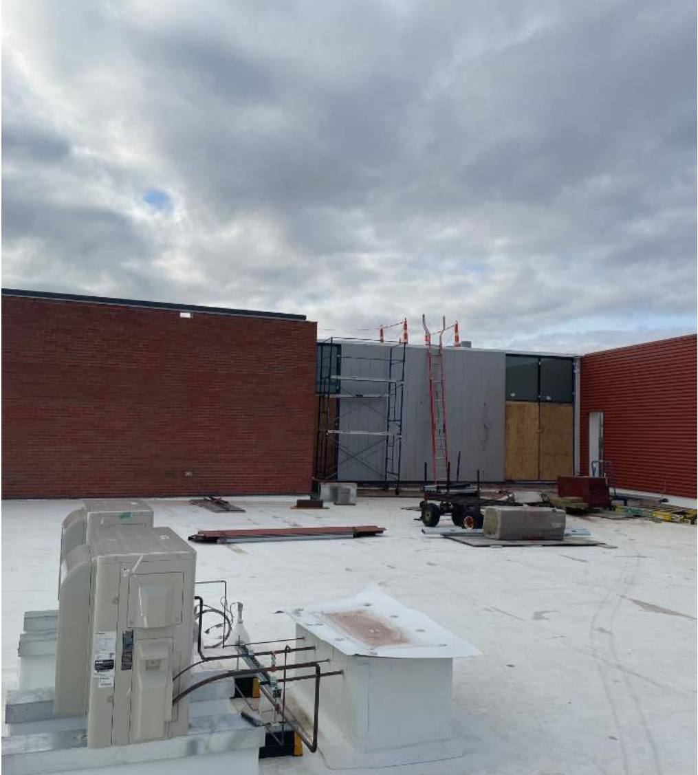
Area D Roof
