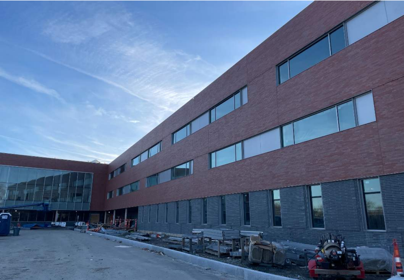
Masonry and Curtain Wall
