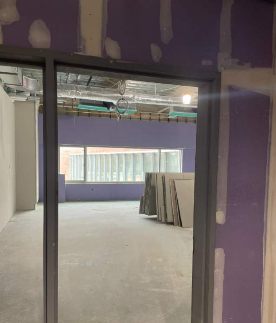
Drywall Finishes and Hollow Metal Frame
