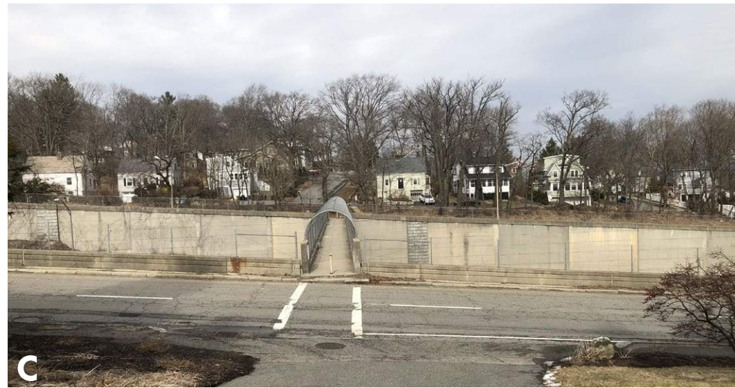
C VIEW OF PEDESTRIAN CROSSING FROM SITE - FACING NORTH
