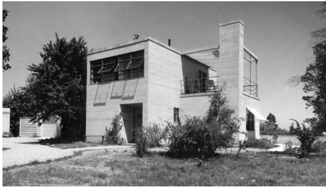
RACHAEL RAYMOND HOUSE - DEMOLISHED
