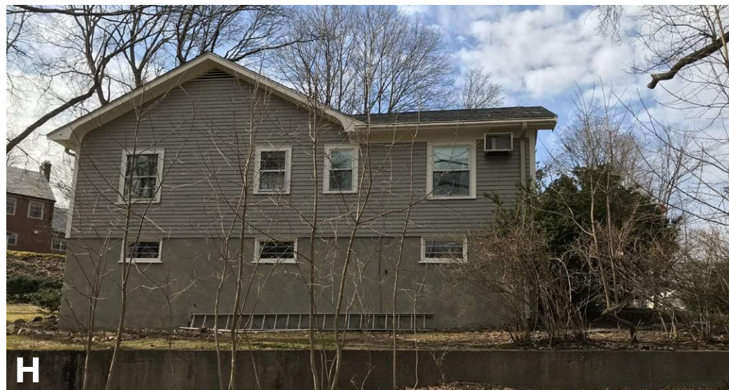
H VIEW OF WEST NEIGHBORING SITE - FACING WEST
