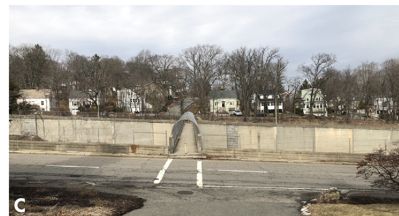
C VIEW OF PEDESTRIAN CROSSING FROM SITE - FACING NORTH
