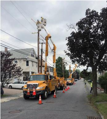
Voltage Conversion Project: Also known as “Project C”, Belmont Light’s voltage conversion project is a long-term initiative to convert existing circuits along with associated equipment and devices from 5kV to 15kV class, thereby enabling us to retire older infrastructure, which correlates to increased reliability.
