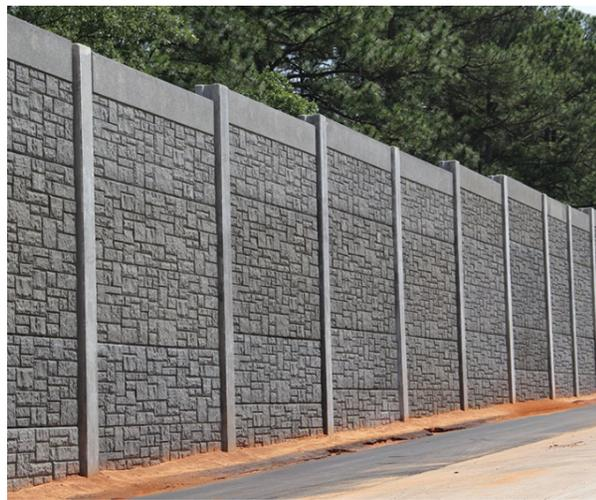
Example Pre-Cast Concrete Vertical Barrier
