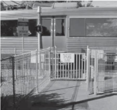
Crossing treatment on the suburban rail network in Perth. Gates automatically close when train is approaching. Users are alerted to the presence of approaching train by flashing lights and audible bells. Gates remain locked until trains have passed. *Perth, Australia*
