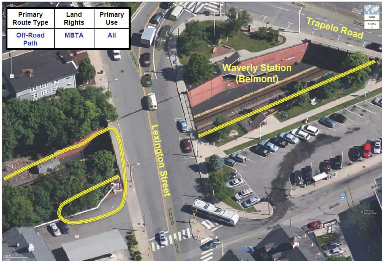
Figure 9-4: Zoom in of Waverley Station for West Belmont MCR Alignment. Proposed wrap-around loop above station platform to avoid busy street crossings.
